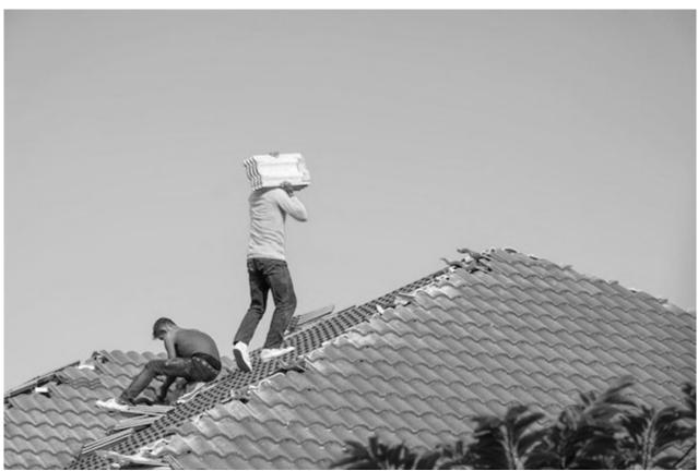
The image shows two workers performing roofing tasks without proper personal protective equipment (PPE). Neither worker is wearing a safety harness, which is crucial for fall protection when working at heights. Additionally, one worker is carrying heavy roof tiles while walking on the sloped roof, increasing the risk of losing balance and falling. The lack of helmets, gloves, and appropriate footwear further increases the danger of serious injuries from slips, trips, and falling debris.
