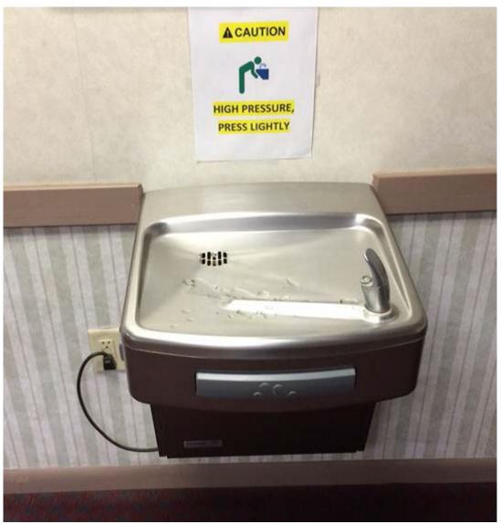
Some people get a charge from energy drinks, but here's a way to get one from a plain old drinking fountain. Notice the position of the plug and outlet, and the sign warning of high-pressure water delivery. And the outlet does not appear to have ground fault circuit interruption (GFCI) protection. Still thirsty? (Naval Safety Center)
