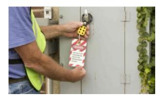
Lockout/tagout particularly applies to any workplace with industrial equipment such as electrical machinery.
