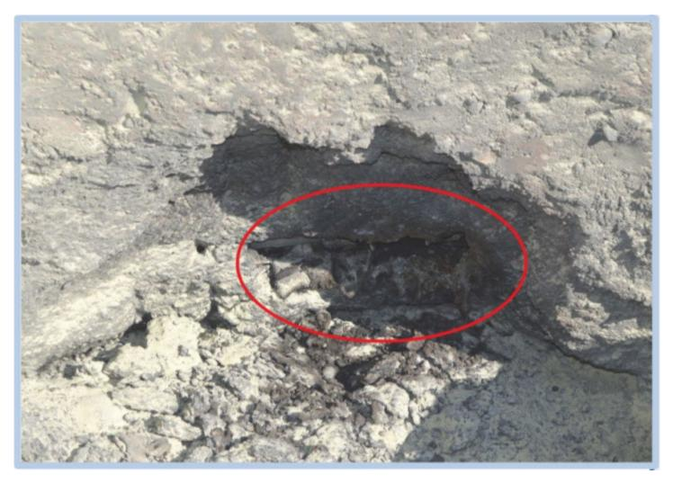
Incident scene where the laborer struck the 7,200-volt power line with his jackhammer as he was chipping away at the concrete encasement of the duct bank.
