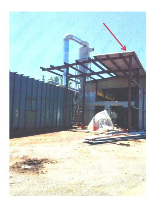
Northeast corner of the roof designated by the red arrow where the victim stepped off the roof falling approximately 24 feet.
